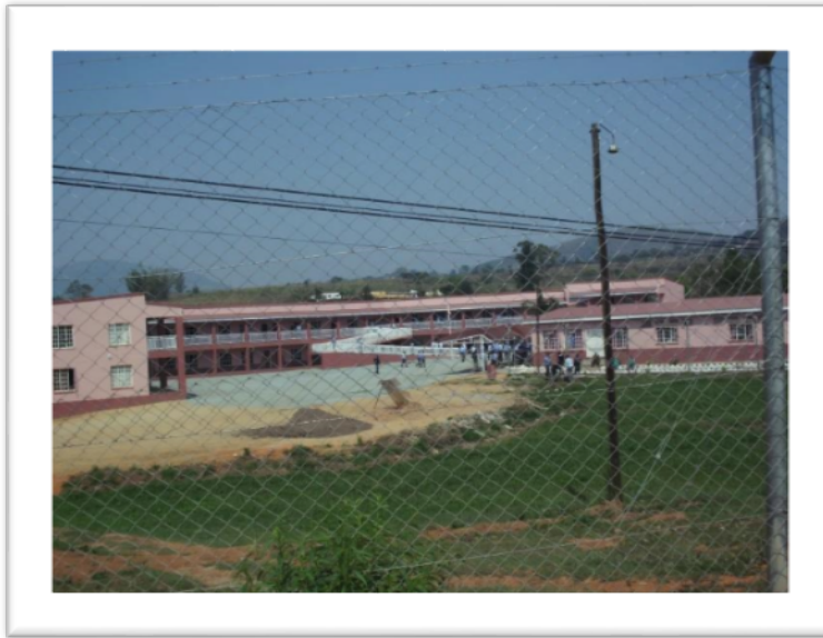
Figure 4: An overview of the school and hostel facility for young male inmates
